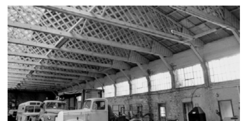
A typical trussed Belfast Hangar.
