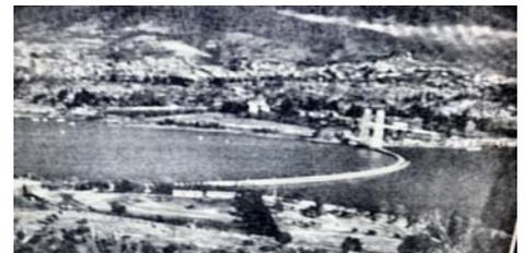
This curved floating bridge was constructed with a series of concrete pontoons weighing a 1,000 tons each. The idea of the curve was to alleviate the need for anchors which were used in straight designs
